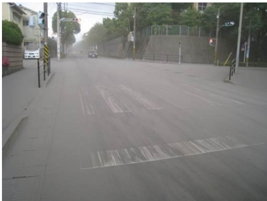
Fig. 8 A road condition that requires clean-up operations (Photo courtesy of Kagoshima City Office)
